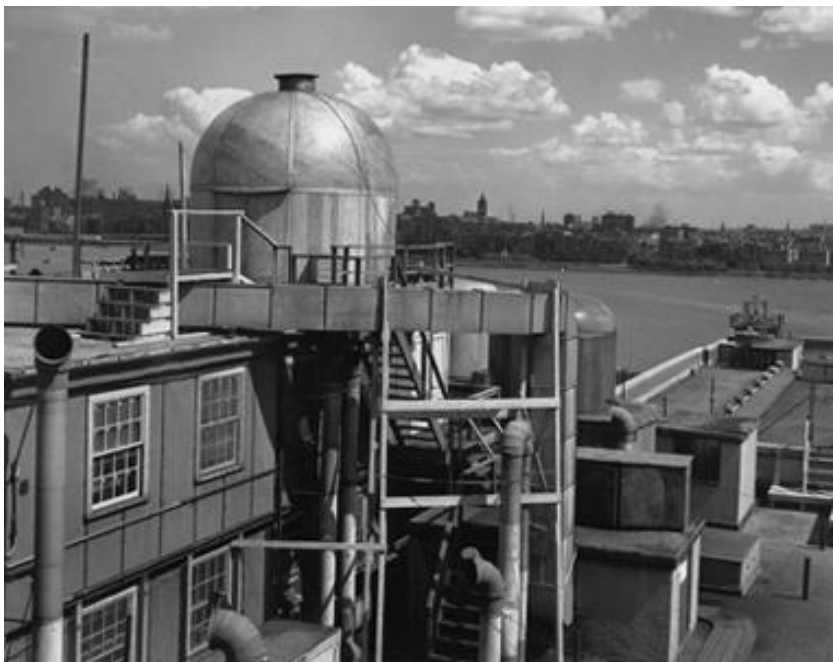
Exhibit 14: Radiation Laboratory Dome, Overlooking Charles River
