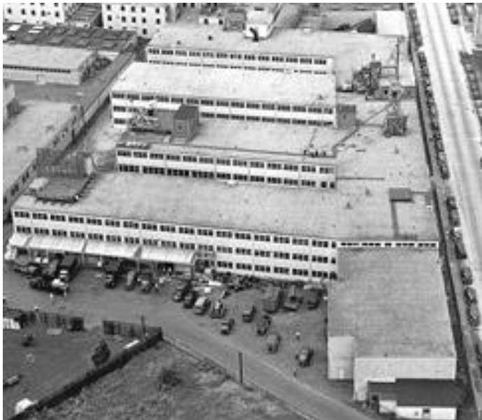
Exhibit 12: Building 20, MIT Campus, Home of Rad Lab from 1943 to 1945
